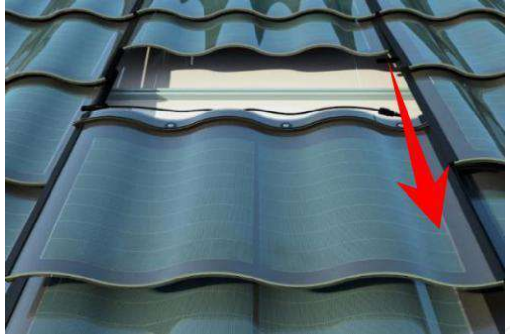
Take off the tile to be replaced
